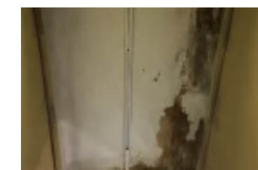
渗漏、腐蚀
